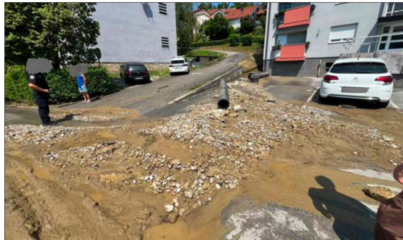
Photogallery: Hole in the ground left by pipe explosion (top left), damage to apartment complex on Gajeva Ulica (top right), debris left behind by water on Gajeva Ulica (bottom).
