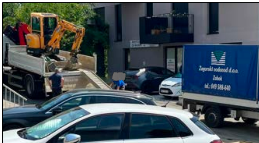
- Zagorski Vodovod on site restoring access to Gajeva Ulica. Photo: Vojtěch Vasiljev
